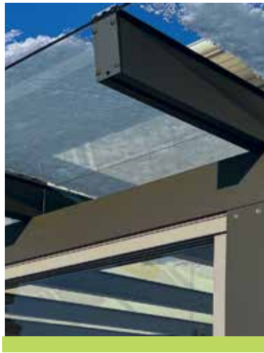
Storm glass between the support beams.
