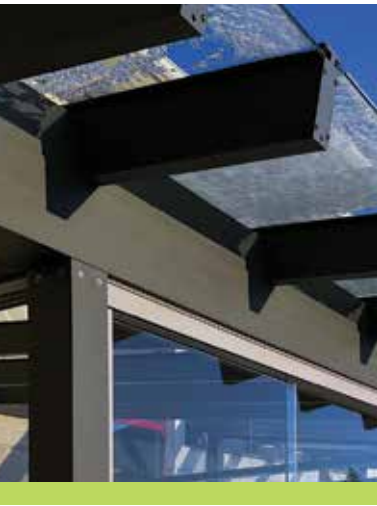
Aluminium storm sheets between the support beams.
